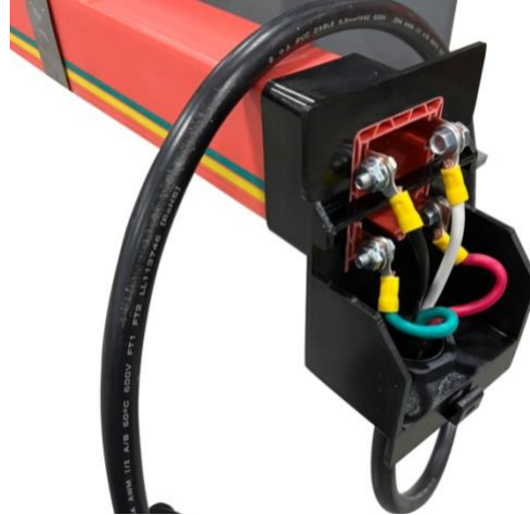
4.6.8 Bolt Head Between the Conductors
