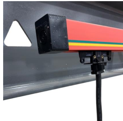
4.6.10 ElectroTrack End Cap Installed
